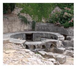
The Castellum Aquae (water basin) was the terminal for the aqueduct in Nîmes. Indeed, the Romans were able to bring to Nîmes water from the source of the River Eure, near Uzès, owing to a 50-km agueduct, of which the Pont du Gard remains the major work that is universally admired.
